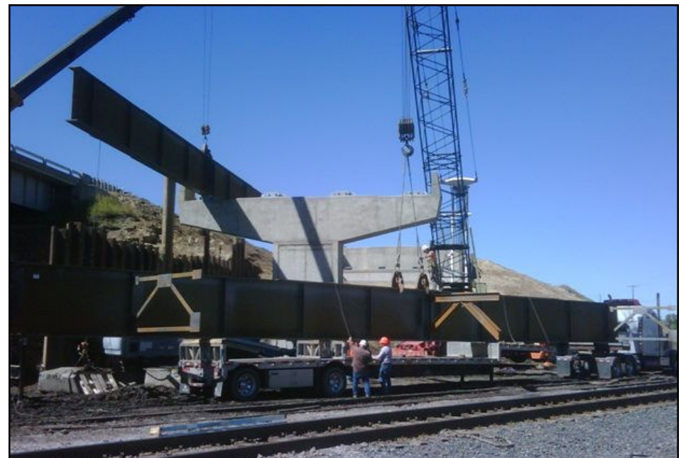
Beam setting, Bozeman Rail Overpass
