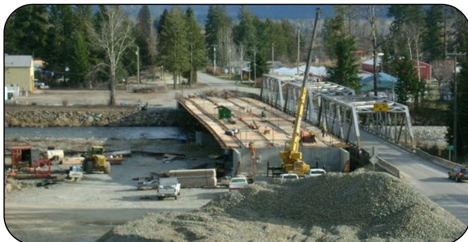
The old and the new Lightning Creek Bridges
