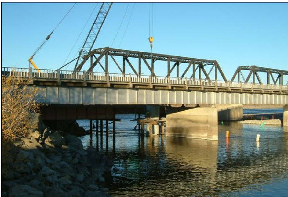
Yellowstone Bridge Rehab at Livingston, Montana
