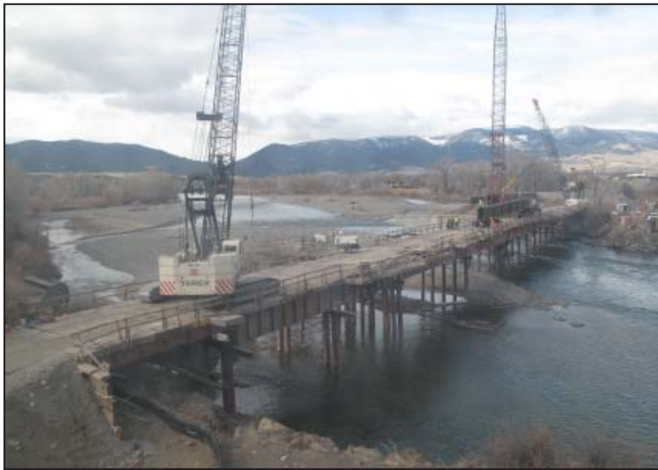
Beam setting at the Yellowstone River Bridge near Livingston, Montana
